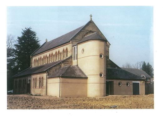
The Chapel has been refurbished and converted to workshop use, whilst sypathetically preserving its historical reference. A first floor and an extension to the rear have been added. The larger workspace the Chapel provides fully meets DEMAND's current needs and allows for future expansion.
